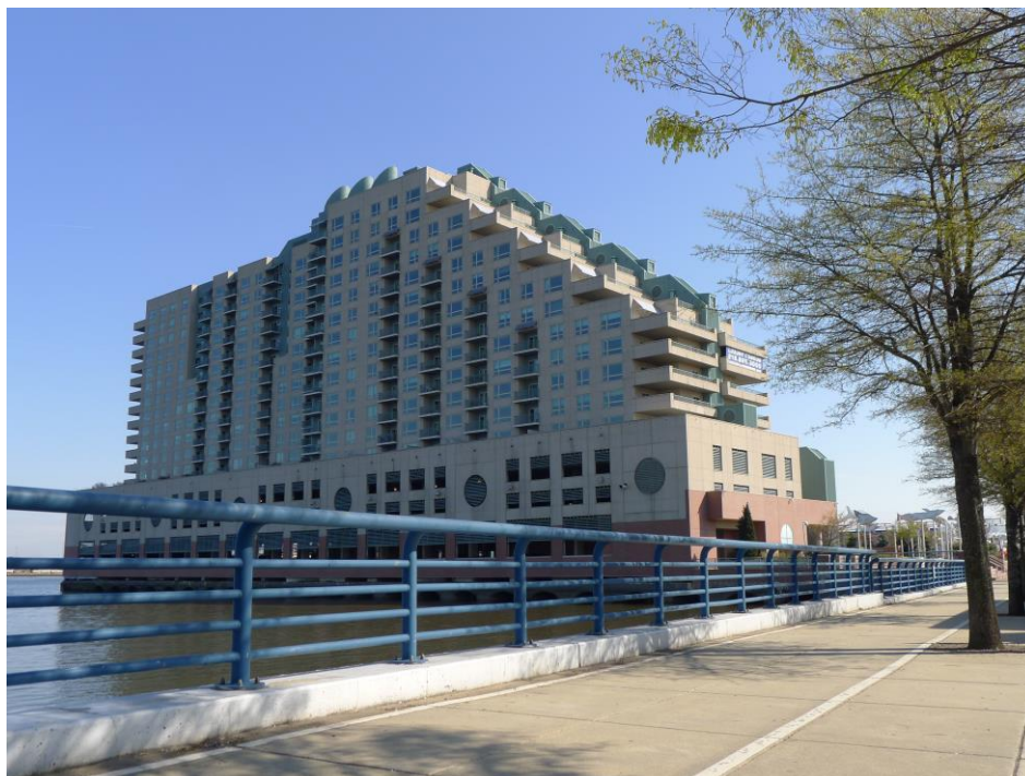
Rys. 1. Dockside Apartments (fot. Łotysz 2012) Fig. 1. Dockside Apartments (phot. Łotysz 2012)
